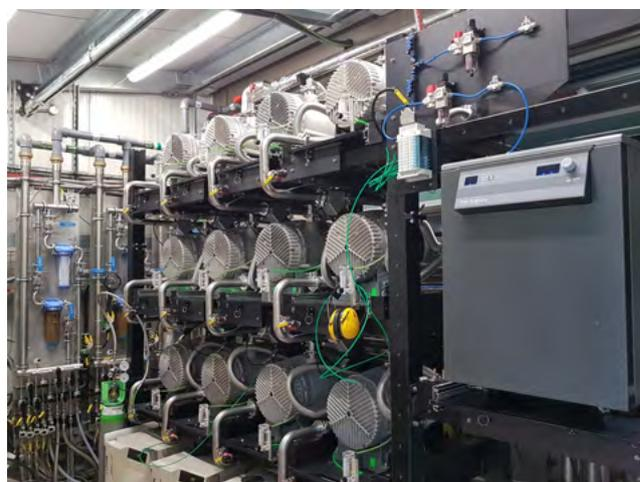
Figure 5: Pumps and compressors are now housed in a separate plant room that opens out onto the back of the building. By segregating these from the experimental stations, we achieve major improvements in noise, and we free up space in the lab.
