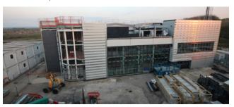
Low carbon concrete has been used, comprising 75% Ground Granulated Blast Furnace Slag (GGBS) instead of traditional Portland Cement. This has reduced the carbon footprint by 48%, saving 1,373 tonnes compared to normal practice.
