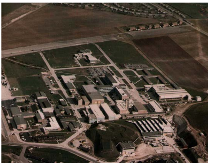
Aerial view of Rutherford Laboratory looking east. In the foreground the green mound of Nimrod, the star shape of the R22 Restaurant is eastwards centre with the houses of Frome Road in the distance. (1963)
