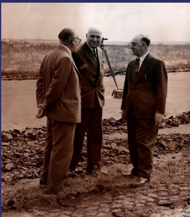
John Cockcroft inspects the Nimrod excavation work. (1957)
