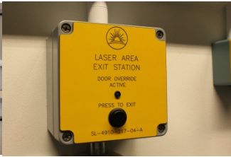
Figure 7 – Entrance door override button
