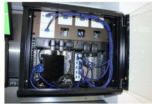
Figure 12 – SCADA equipment panel containing PC and VGA distribution units
