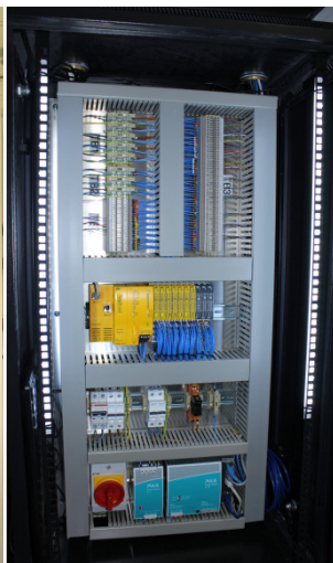
Figure 9 – Main safety panel containing the new PSS4000
