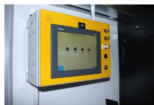
Figure 4 - HMI Panel for laser control
