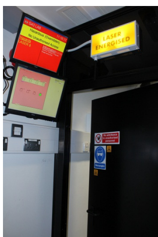
Figure 11 – Lab entrance hazard/information screens showing single laser hazard present. Door has been overridden to enter lab
