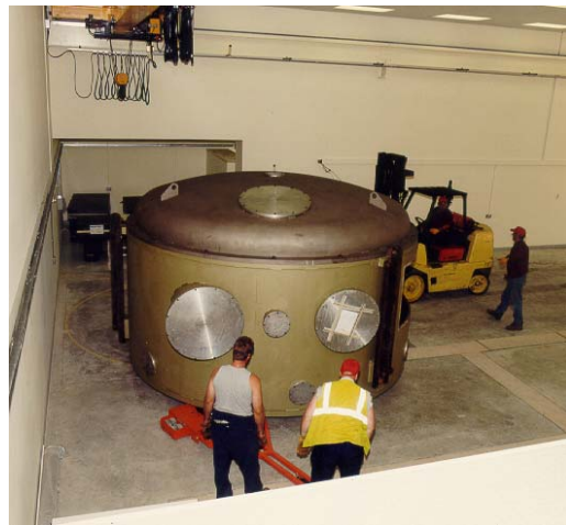
Photo 2. The north tank of the compressor chamber being positioned inside the target area.
