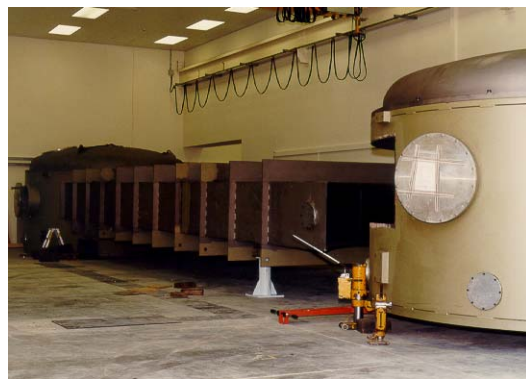
Photo 4. The interconnecting tunnel of the compressor chamber being positioned between the two tanks.
