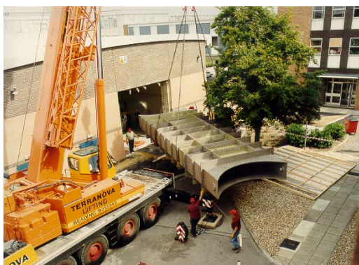
Photo 3. The interconnecting tunnel of the compressor vessel being brought into the building.
