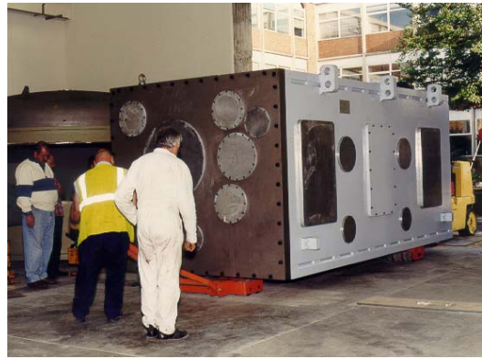
Photo 6. The interaction chamber being positioned in the target area.
