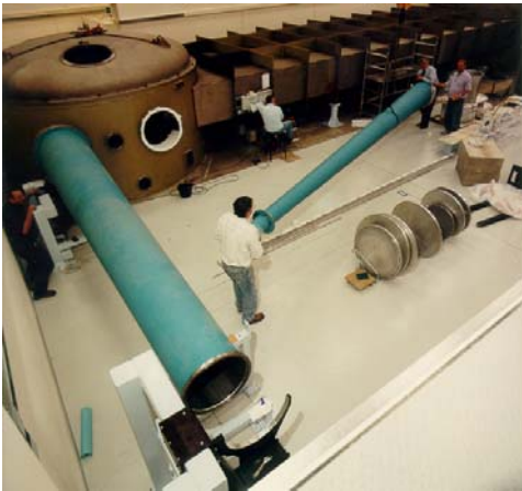
Photo 7. The vacuum spatial filter tubes being assembled.
