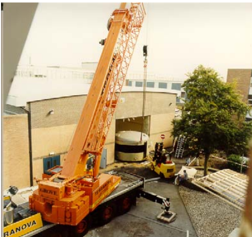
Photo 1. The north tank of the compressor chamber being brought into the building.
