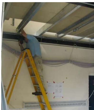
Figures 3, 4 & 5. installing stairs at ground floor level between Laser Control Room and new Target Area 2 Control Room, installing the mezzanine and ceiling above the new Target Area 2 Control Room.
