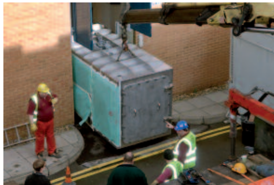
Figure 8. Quinto deliver compression chamber into south control room 29/2/08.
