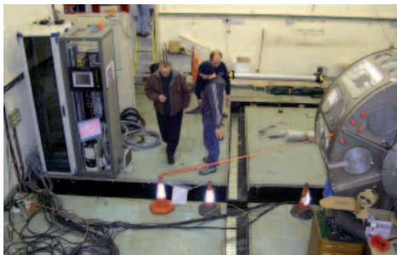
Figure 5. Changing booth removed and trenches open.
