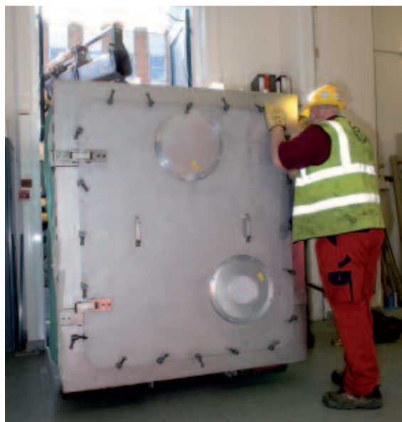
Figure 7. The new compression chamber enters the south control room.
