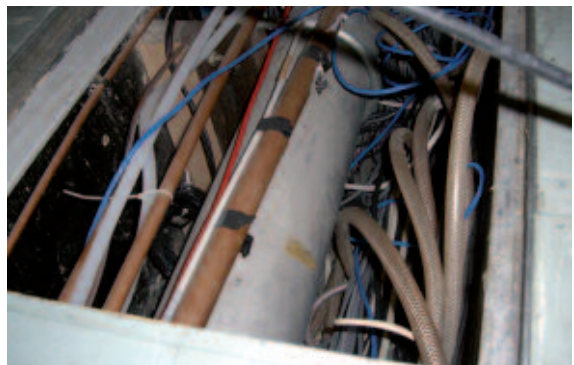
Figure 3. Existing TAW trenches.
