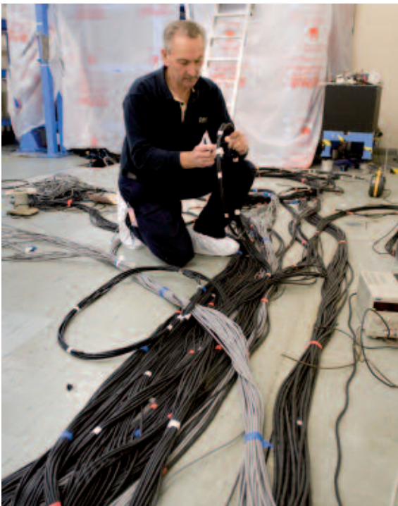
Figure 11. First batch of drive cables are installed.
