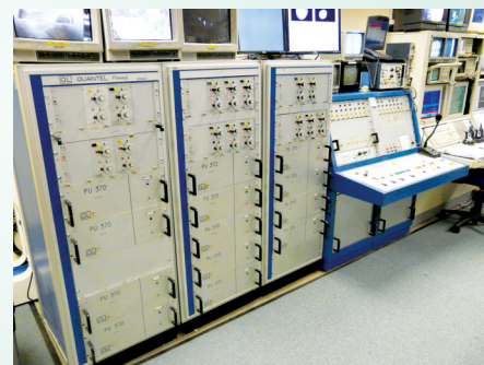
Old Quantel units inside the Vulcan Main Control Room.
