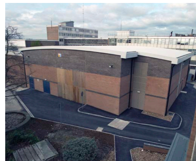
Finished Vulcan Petawatt building, 2001. (01RC1105)
