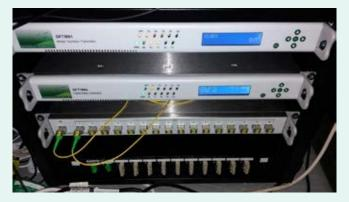
Installation of the Greenfield Master Oscillator and Slave Unit in the Front-End Oscillator Room.
