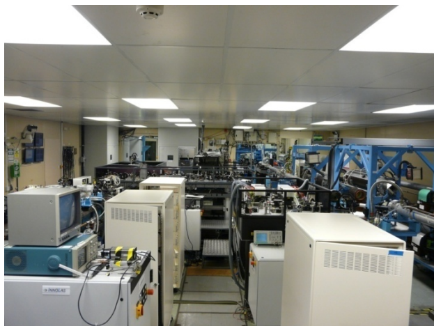
Figure 4 – Laser Area 1 with new Quantel hardware installed.
