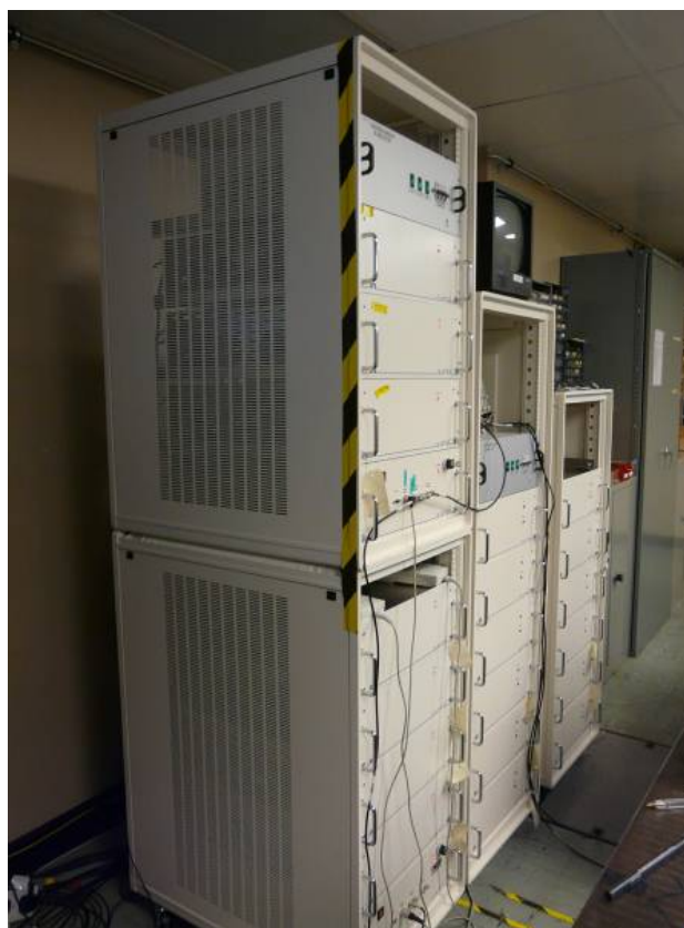
Figure 5 – New Quantel racks, located on north wall of Laser Area 1, to power the 45mm rod amplifiers and control processing and power of both rod chains.
